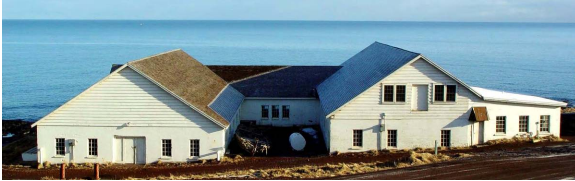
Figure 3. The St. George Sealing Plant was designated a National Historic Landmark building in 1962. It was recently the focus of a $2 million renovation project to preserve the plant's structural and historical integrity. The restoration was completed in 1999 by the St. George Tanaq Corporation and NOAA.
